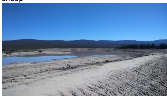
Plate 4: Earth-wall dam with water
