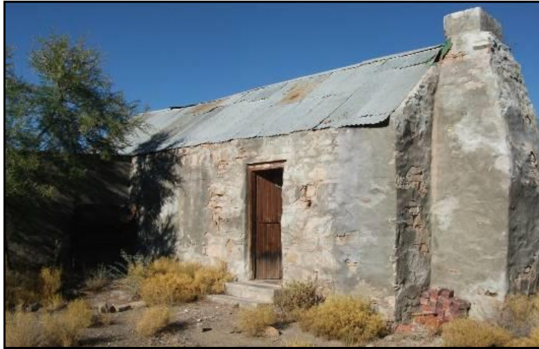
Plate 3: The abandoned farmhouse at Wolven Hoek, which probably dates to the late 19 th century, has been partly restored. It is older than 60 years and protected in terms of the NHRA. It is located within 2m of the farm access road.
