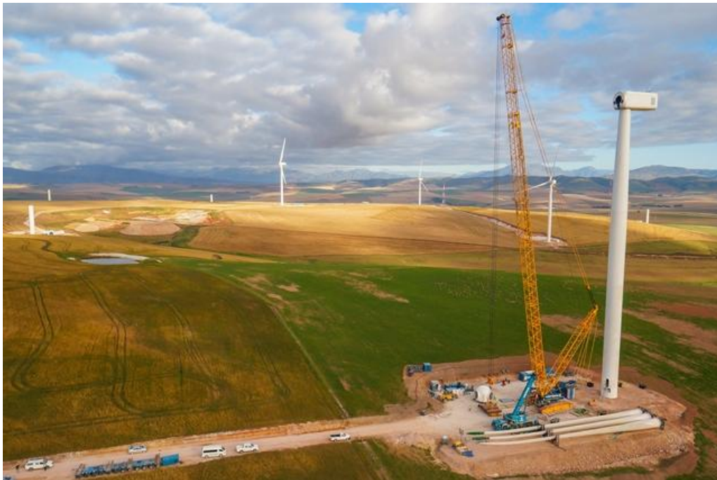
Figure 3 Example of turbine construction
