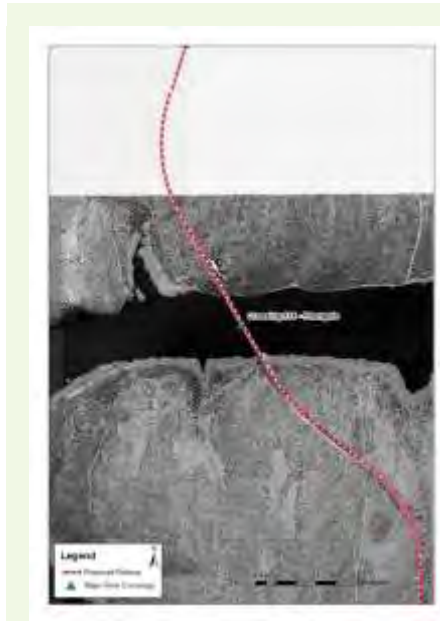
Figure 75: Aerial view Phongolo River crossing
