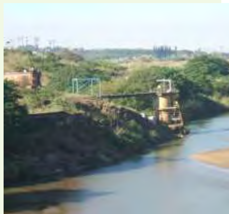
Figure 34: Abstraction 400m downstream of existing bridge
