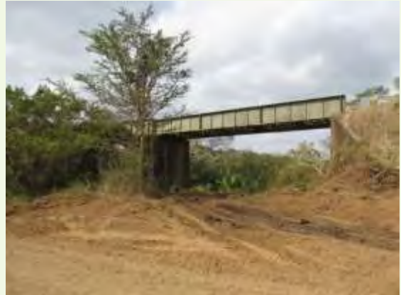
Figure 46: Existing Mzinene bridge
