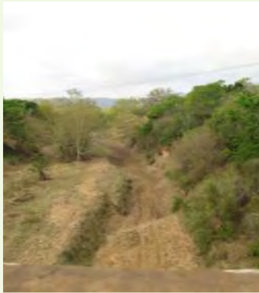
Figure 64: Looking downstream Msunduzi crossing
