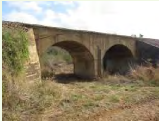
Figure 54: Existing Mhlongisa bridge
