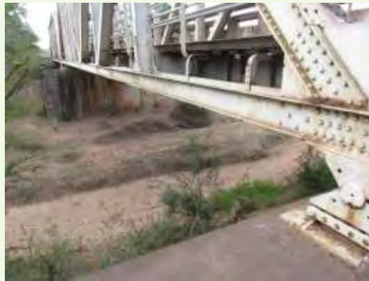
Figure 62: Existing Msunduzi bridge.
