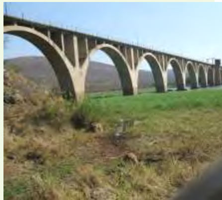
Figure 76: Existing Phongolo bridge
