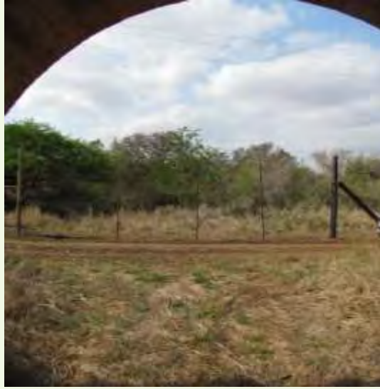
Figure 56: Looking downstream at Mhlongisa crossing
