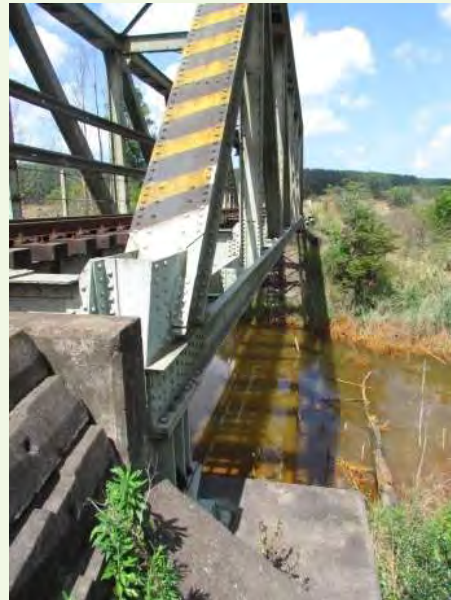
Figure 27: Existing Mposa River Bridge
