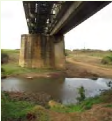
Figure 41: Existing Hluhluwe bridge
