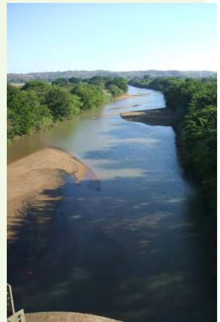
Figure 35: Mfolozi crossing upstream of existing bridge
