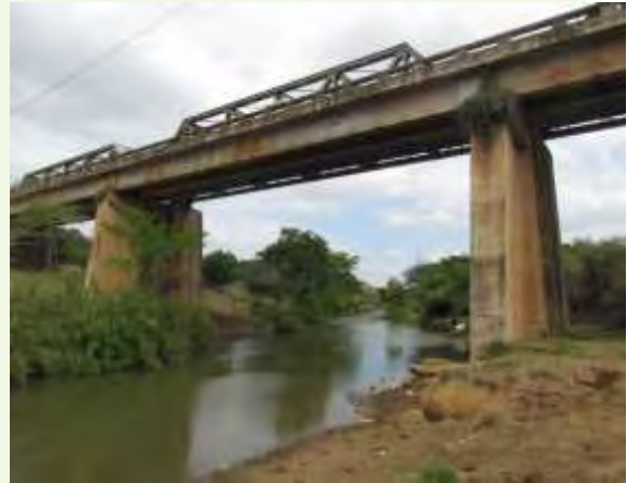
Figure 37: Existing Nyalazi bridge
