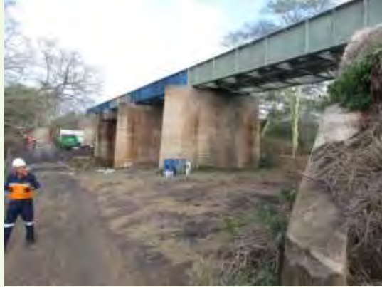
Figure 58: Existing Mduna River bridge
