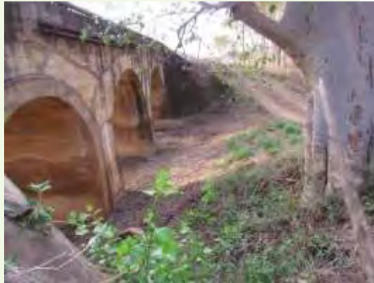
Figure 66: Existing KwaSekene bridge
