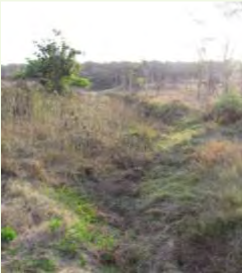
Figure 67: Looking upstream KwaSekene crossing
