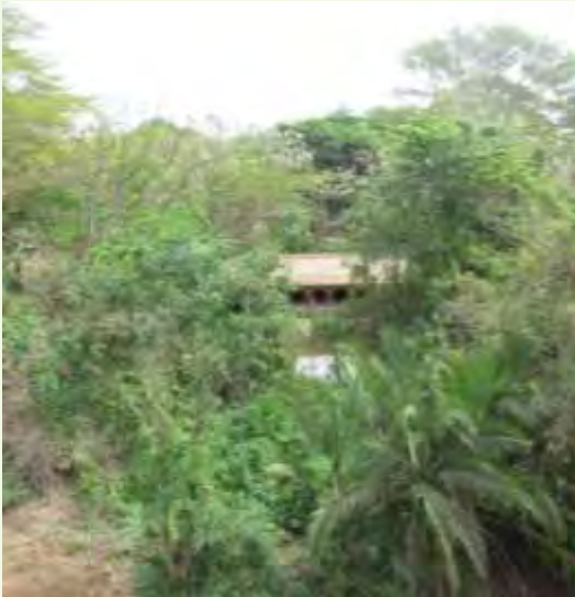
Figure 51: Looking upstream at Ngweni crossing
