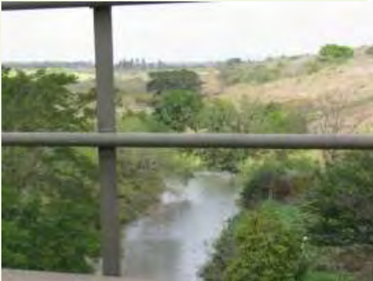
Figure 38: Looking upstream Nyalazi crossing
