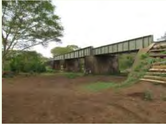
Figure 50: Existing Ngweni Bridge
