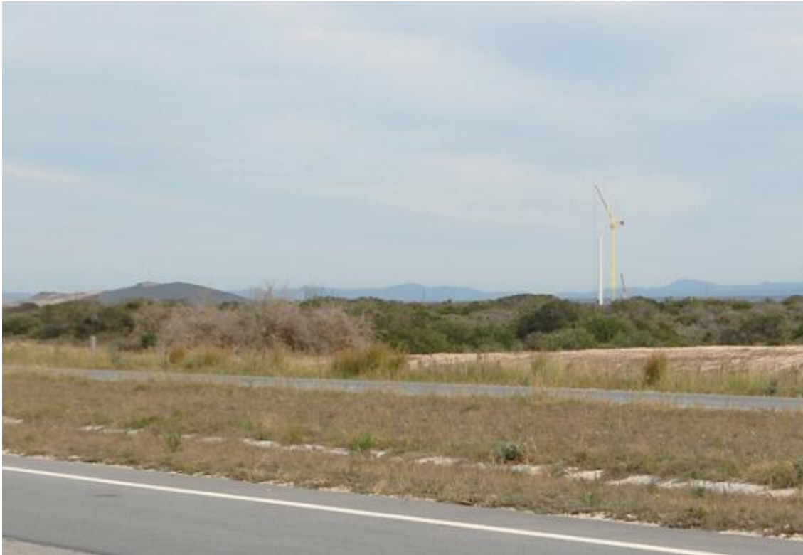
Plate 9-1: Construction of the existing Coega wind turbine
