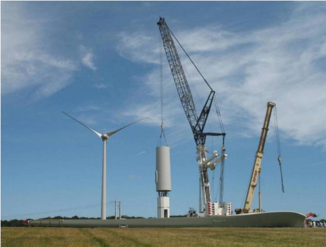
Figure 2-5: Assembly and erection of the tower sections
