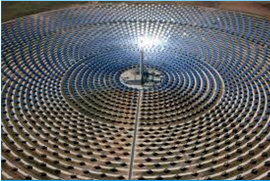
Figure 1-3: Elliptical formation of the Central Tower Solar Field
