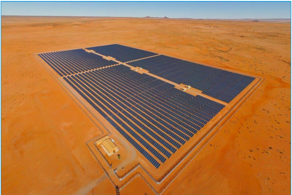
Figure 1-5: Large-Scale Photovoltaic Power Generation Facility
