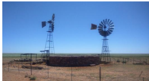
Plate 4 – Windmill-driven boreholes and reservoir
