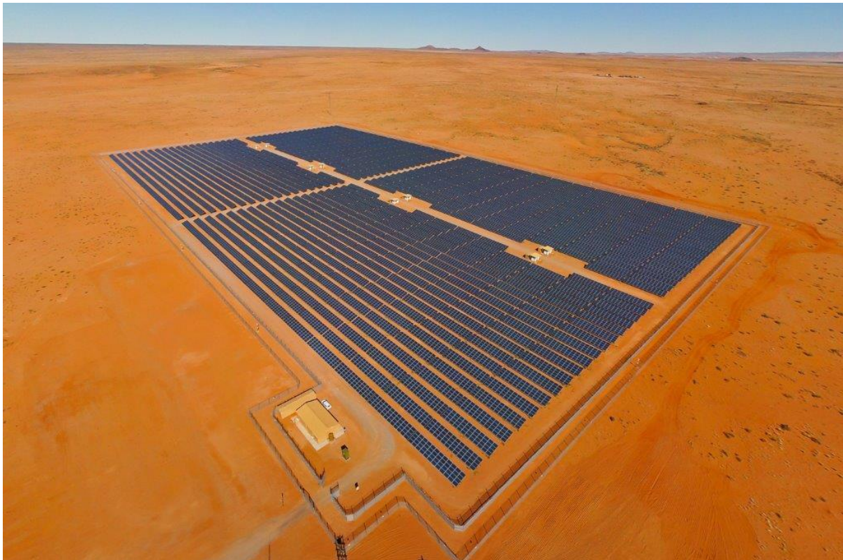
Plate i: Large-Scale PV Facility (Source: www.pv-magazine.com )
