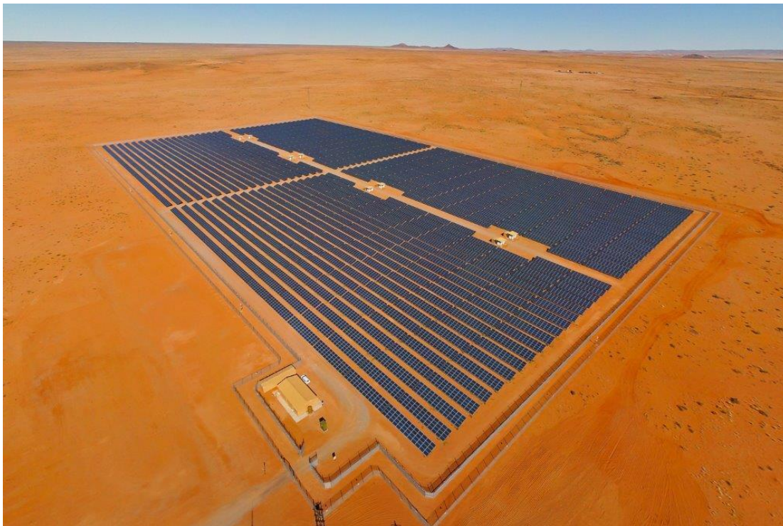
Plate i: Large-Scale PV Facility (Source: www.pv-magazine.com )
