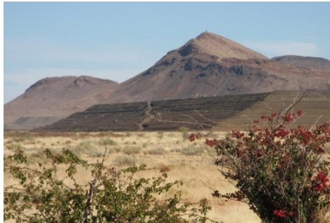
Plate vii: Mining: Black Mountain tailings dam
