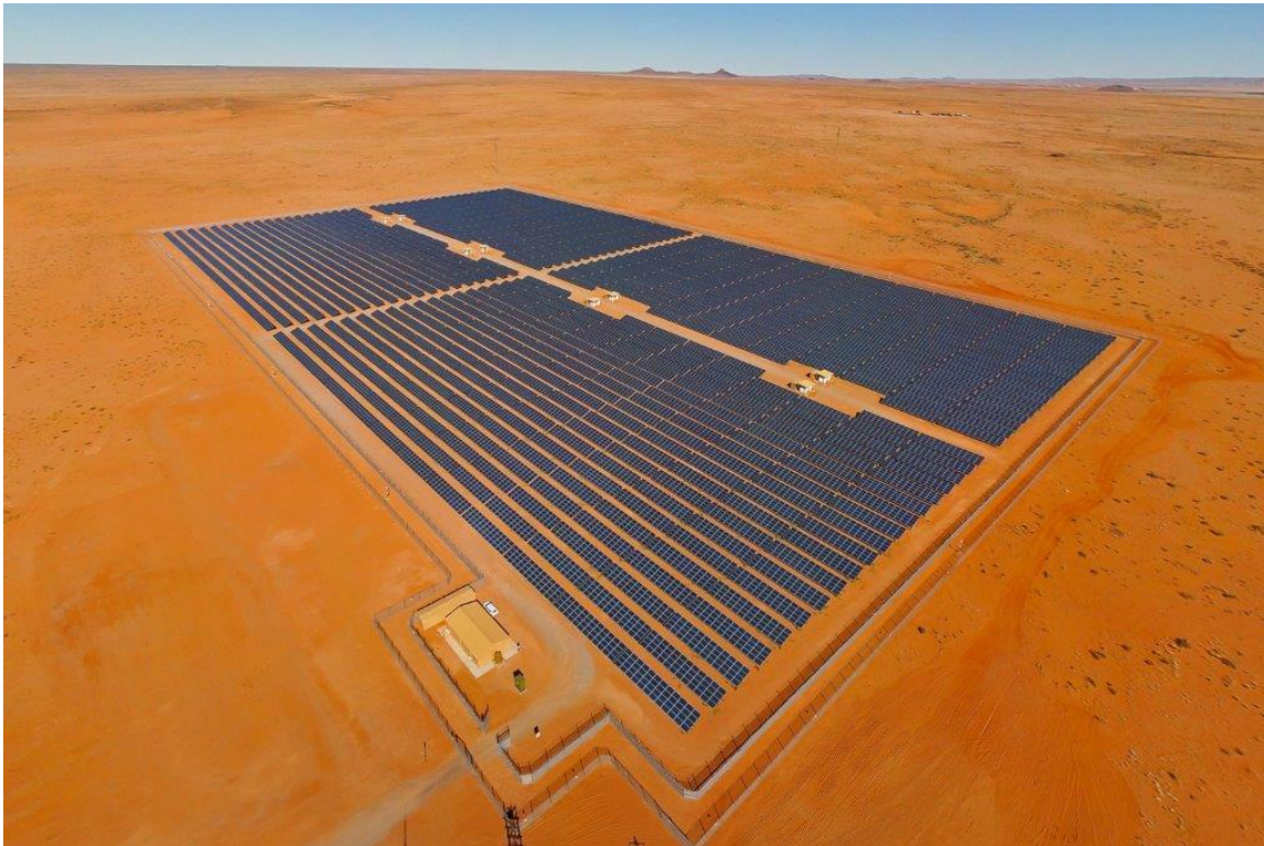
Plate i: Large-Scale PV Facility (Source: www.pv-magazine.com )
