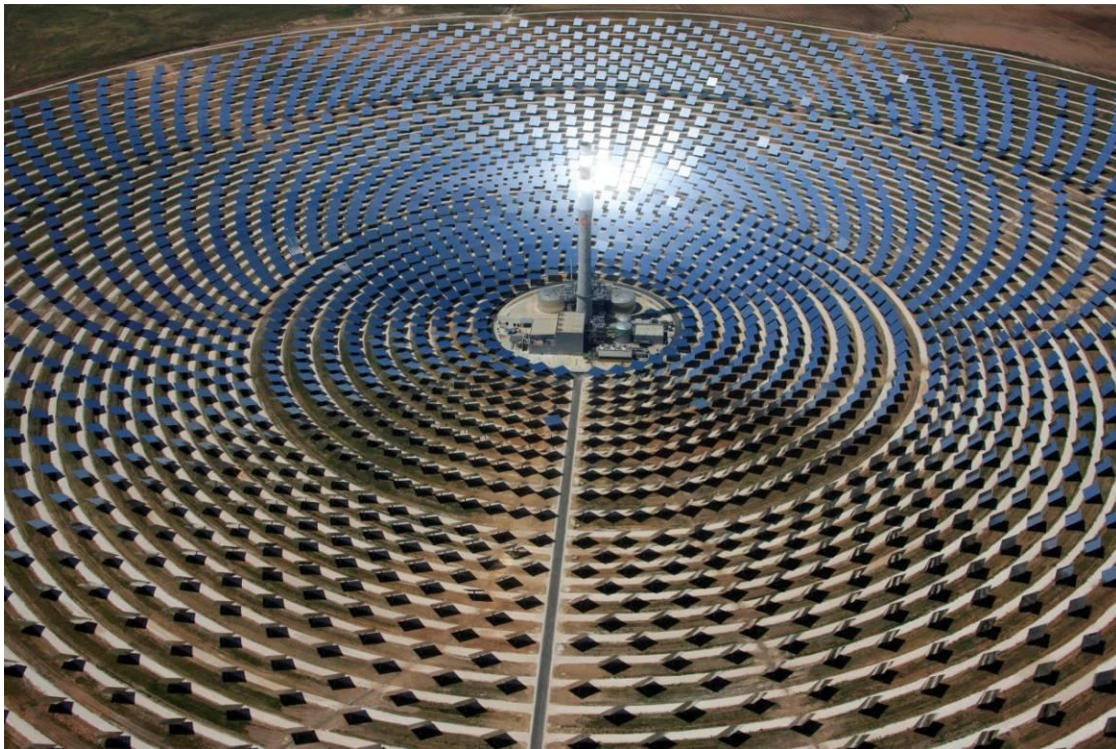
Plate ii: Elliptical formation of the Central Tower Solar Field (Source: www.finetubes.co.uk )
