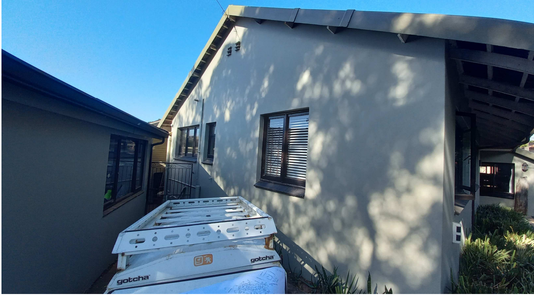
(Authors Picture) LEFT VIEW OF BUILDING (GOOGLE EARTH) ARIEL SITE:
