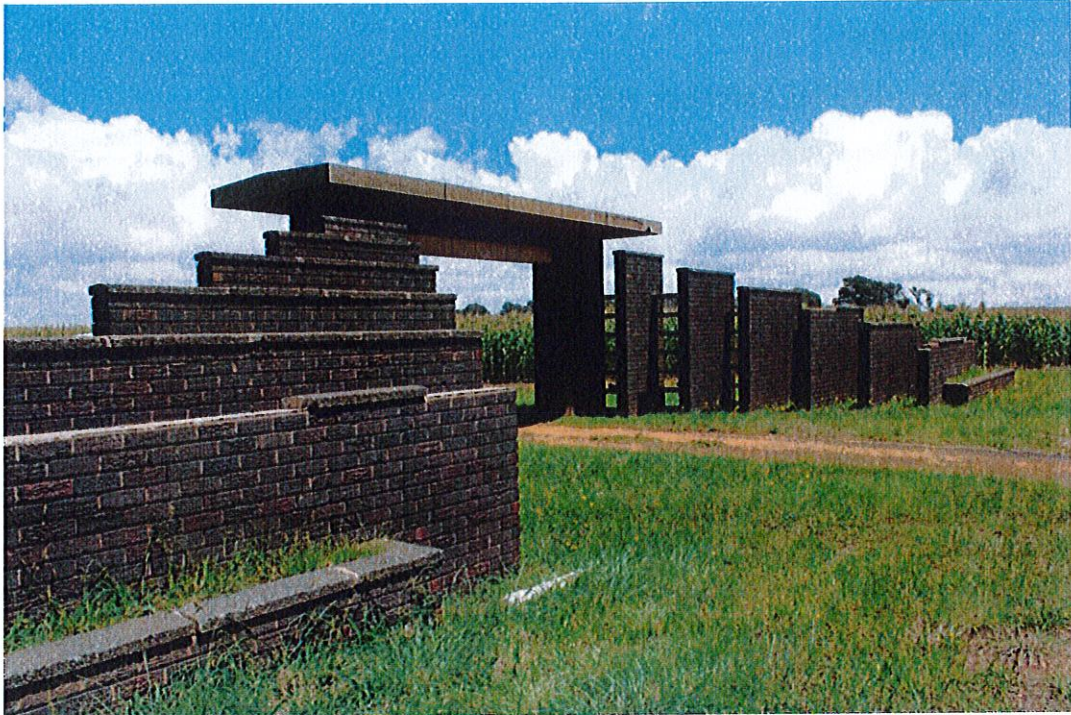
Figure 16: Area earmarked for development. Proposed widening of the N4 along section 5B between Belfast and Machado Toll Plaza. Bergendal Monument entrance gate.
