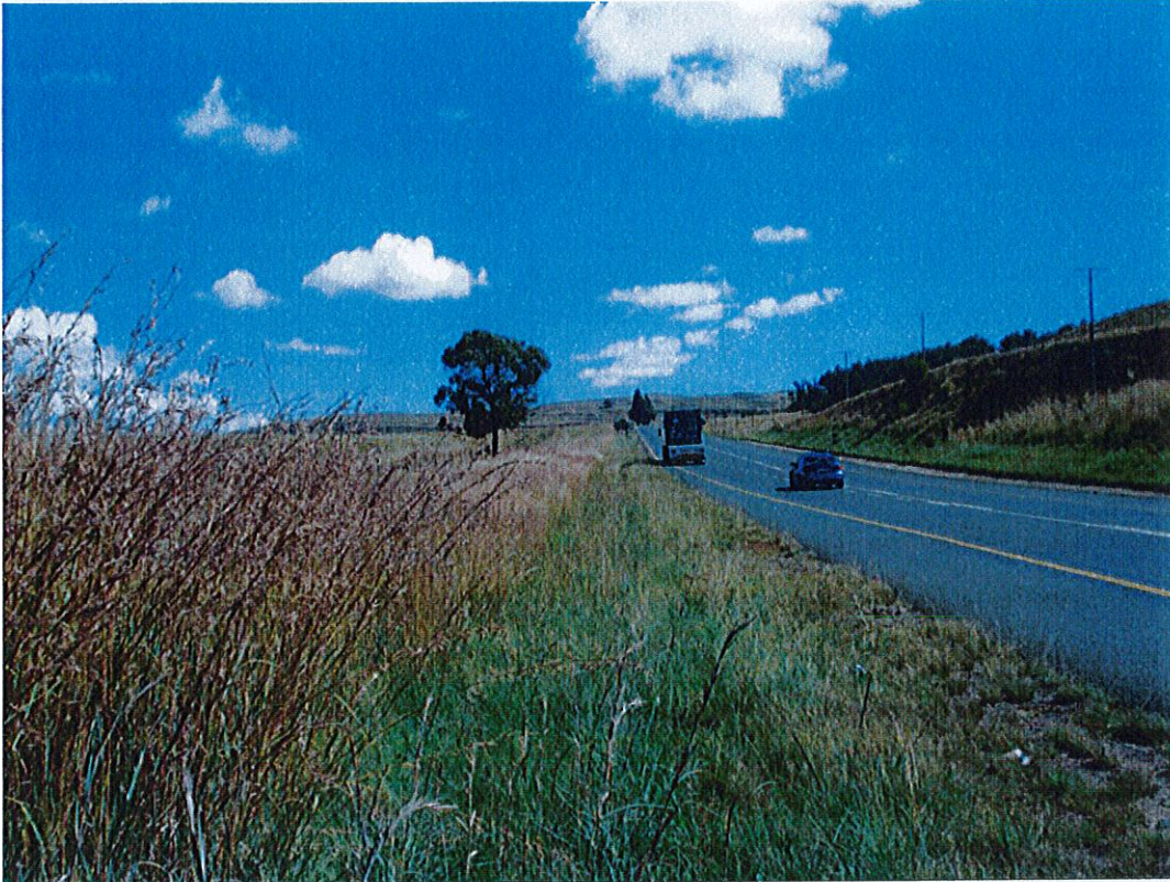
Figure 13: Area earmarked for development. Proposed widening of the N4 along section 5B between Belfast and Machado Toll Plaza.
