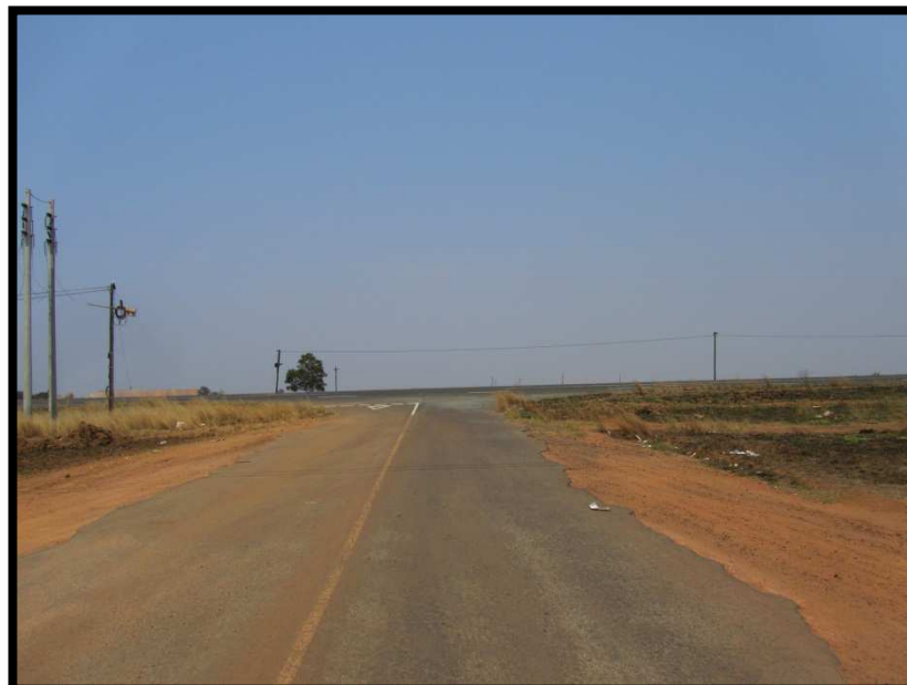
Figure 2: Access onto R544
