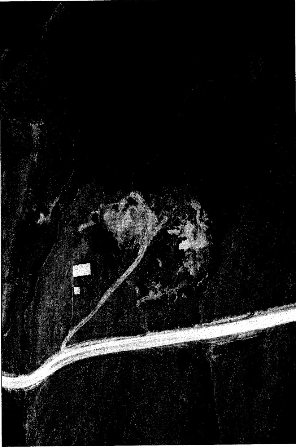
View of the borrow pit from the air
