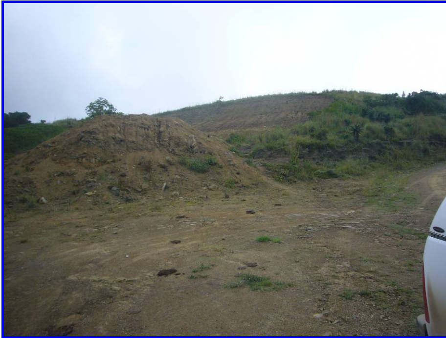
Figure 25: Borrow Pit # 348-BP03.
