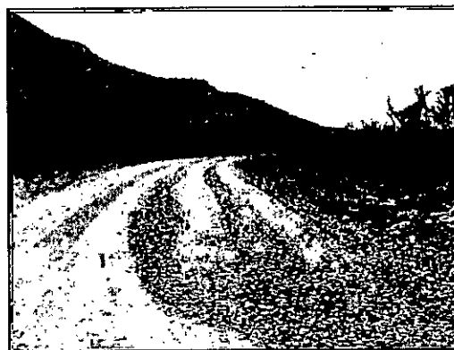
Figure 40: Upgrading of Road nr 654 in progress
