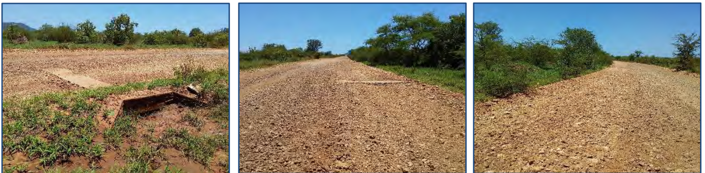
Figure 2-4: Water Crossing A: view from the horizontal alignment of the road
