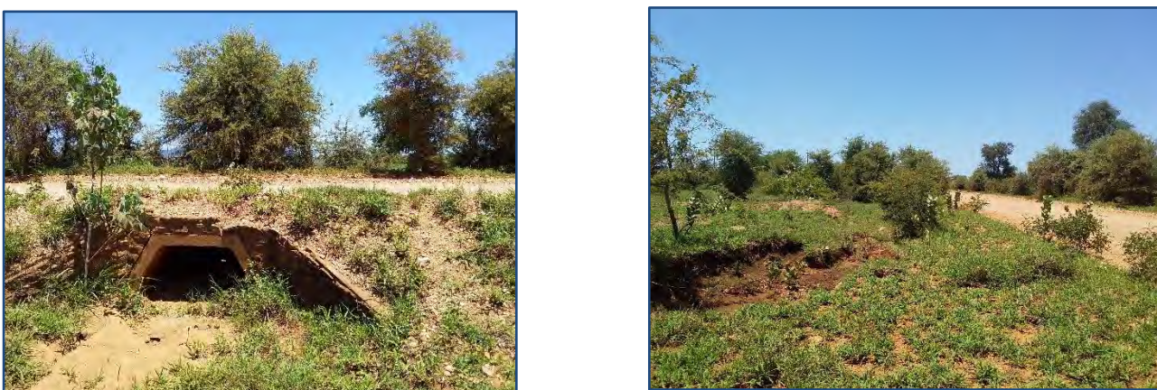
Figure 2-5: Water Crossing B: View from the horizontal alignment of the road
