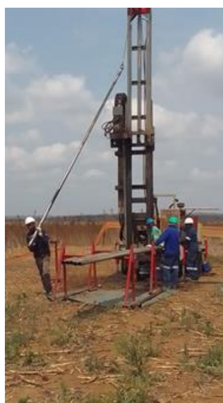
Figure 10: Example of the drilling machinery
