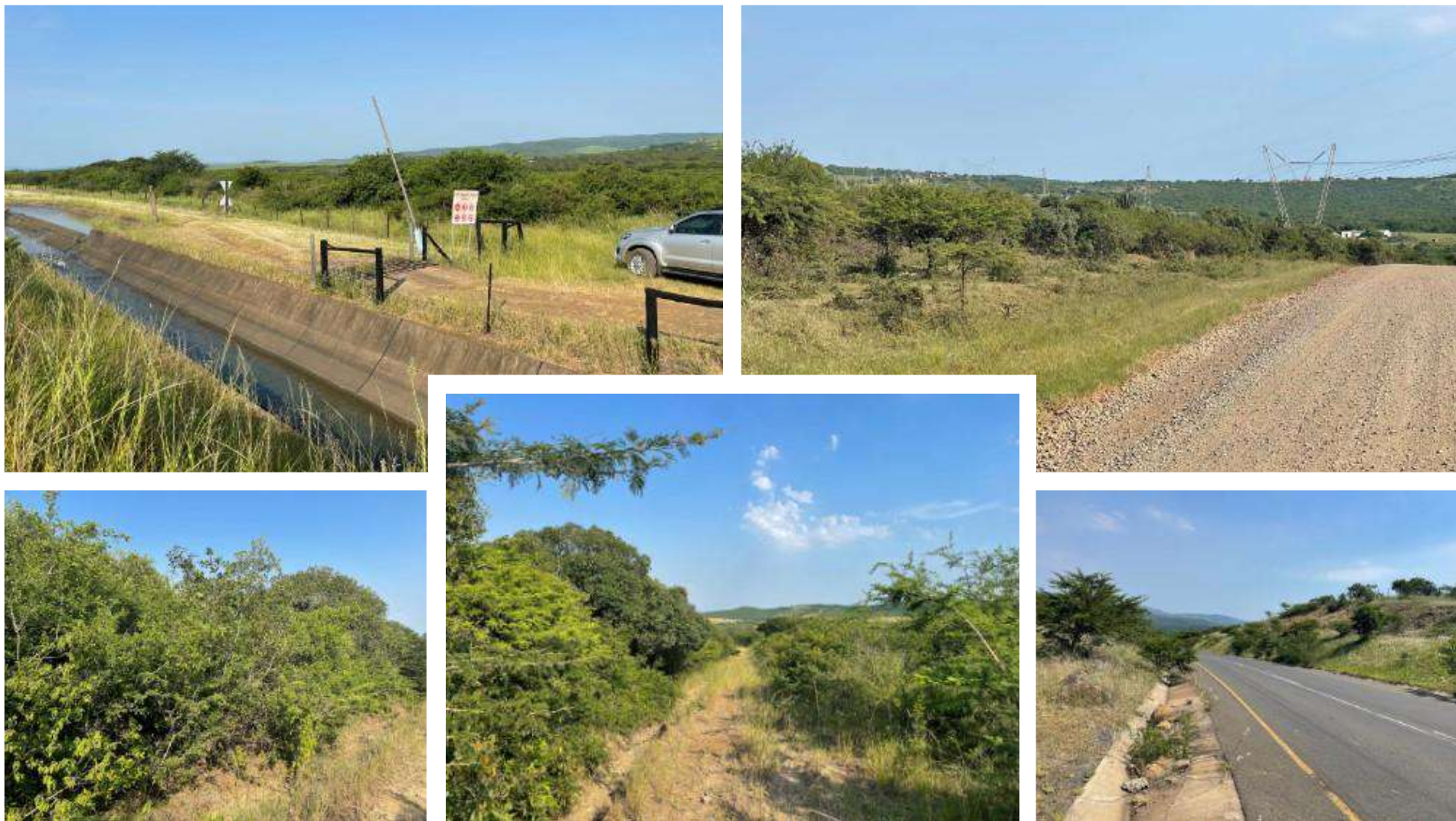
Figure 7: Overview of Point 38-30, the servitude is dominated by indigenous plant species.
