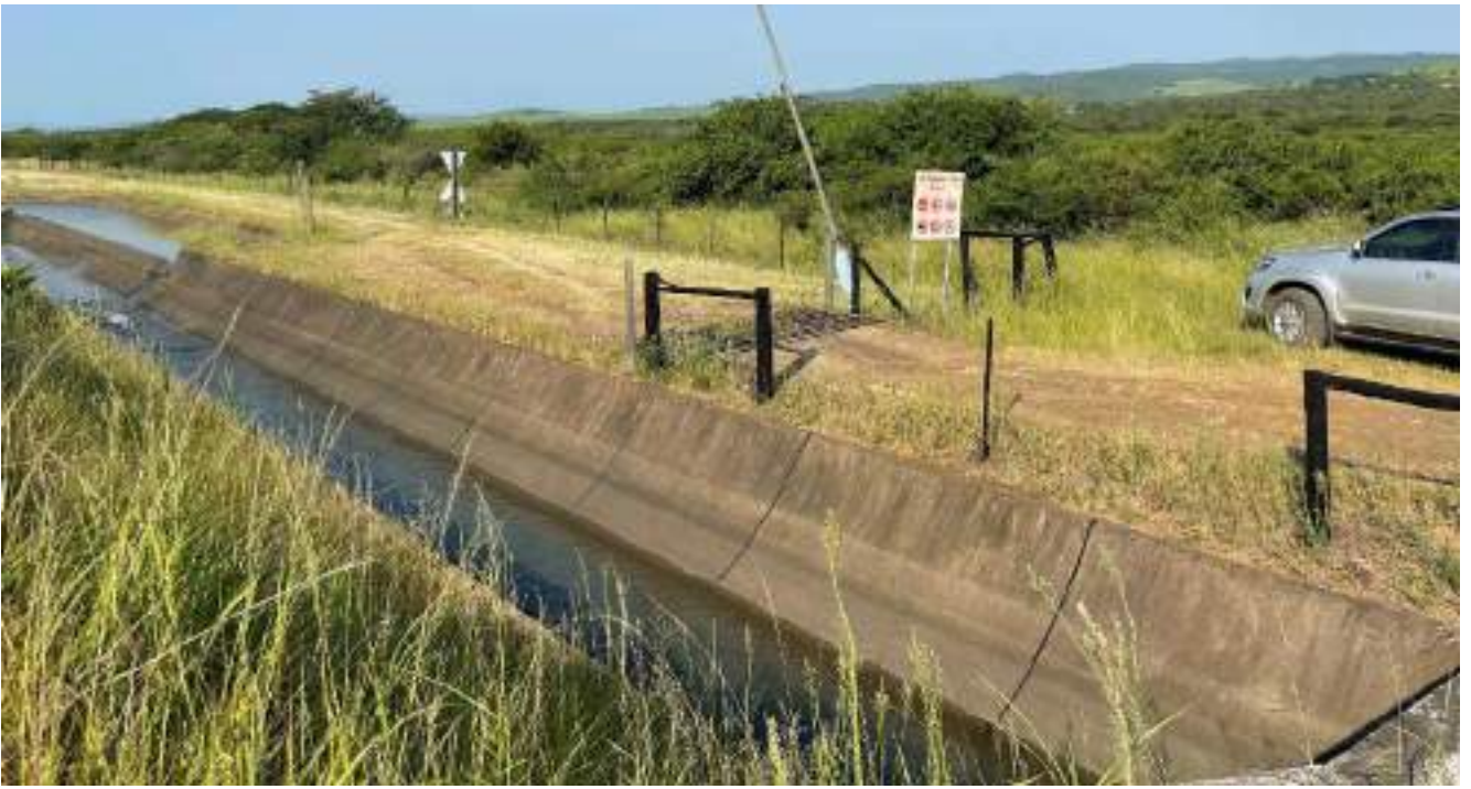
Plate 14: showing agriculture infrastructure within the proposed project area
