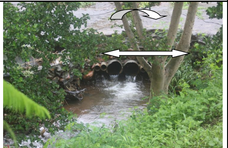
Figure 16: Existing bridge crossing on the eastern drainage line.
