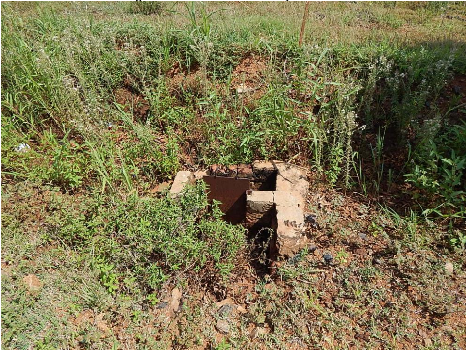
Fig. 14: Several sluices are visible within the earth canal to regulate water, on the study area.
