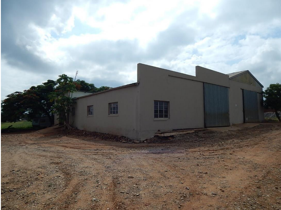
Fig. 25: The farm sheds in the north, and near the banks of the Crocodile River.
