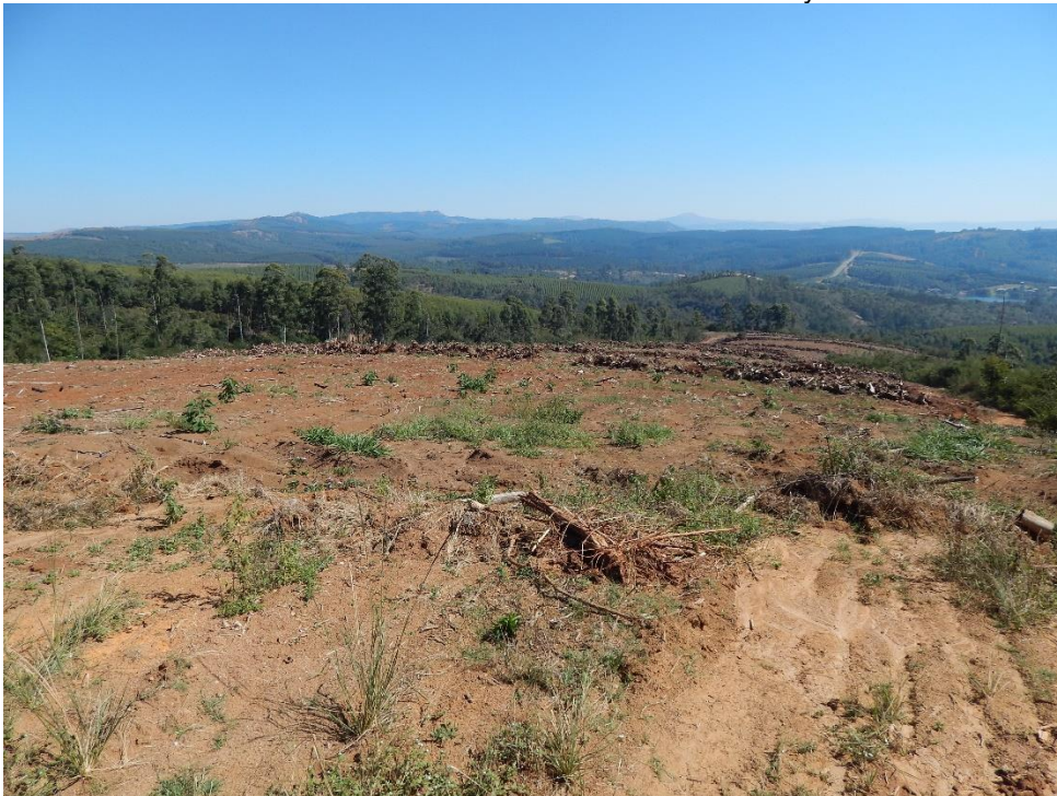
Fig. 2: The area for Dam 1 was previously a timber plantation which has been cleared of vegetation. The view faces north.
