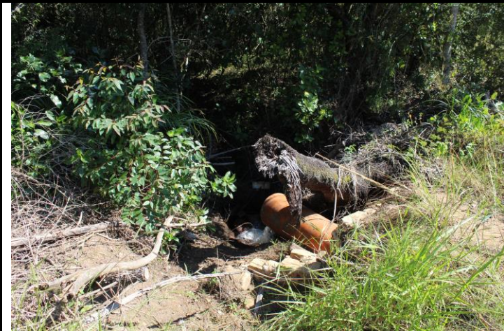
Figure 19: Weir 1: Drainage line outflow.
