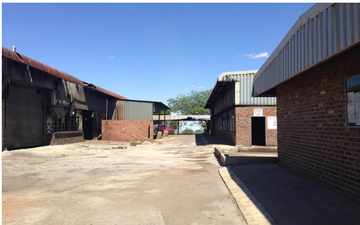
Figure 7: Existing buildings (building 3 at the back on the right of the photograph)
