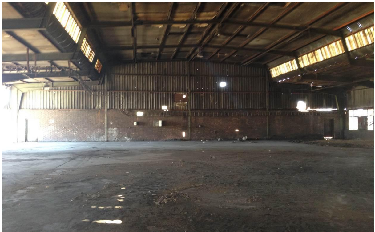
Figure 9: Inside of building 2
