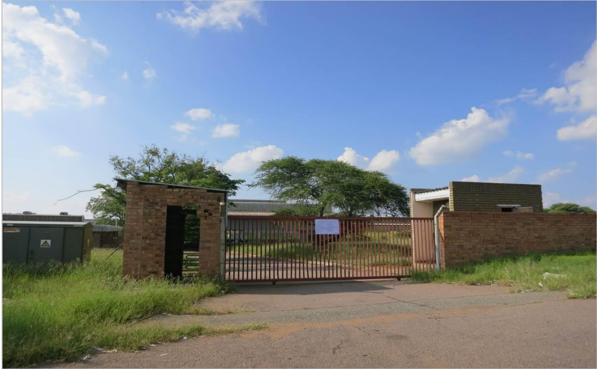
Figure 26: Site notice 1 at the entrance gate to the proposed site
