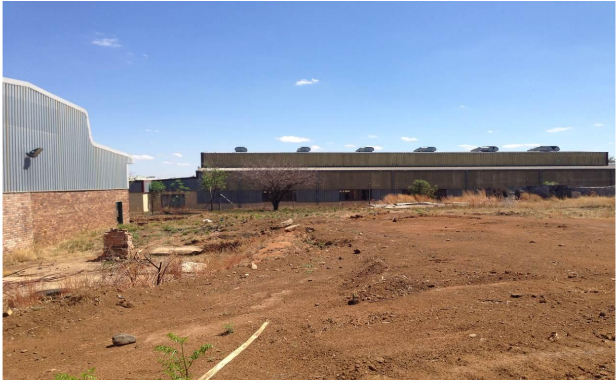
Figure 12: Open piece of land to the east of the three existing buildings (2)
