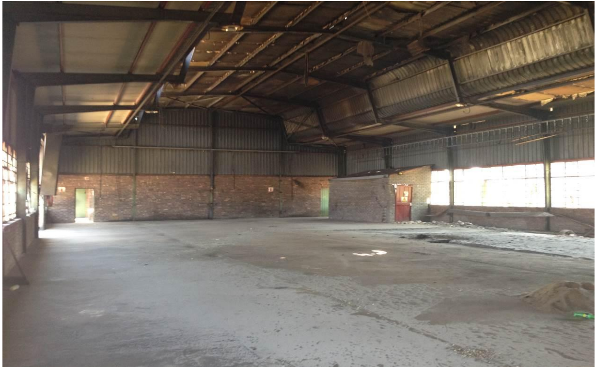
Figure 10: Inside of building 3
