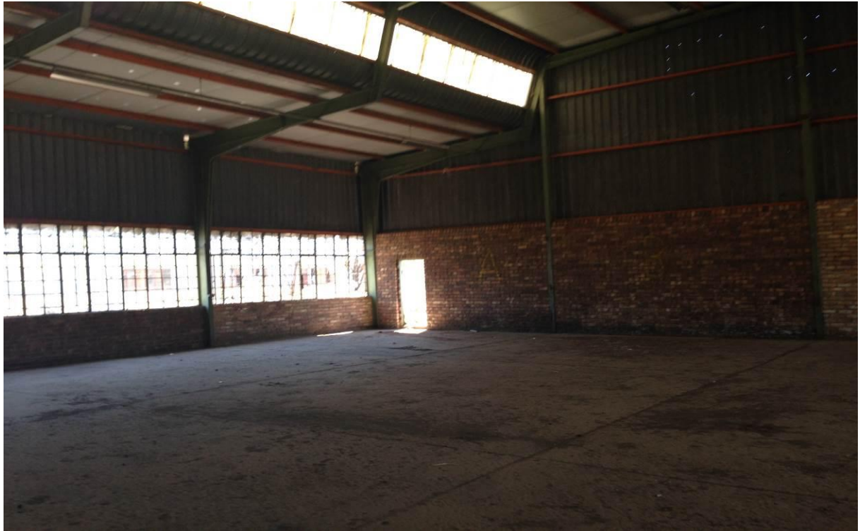
Figure 8: Inside of building 1
