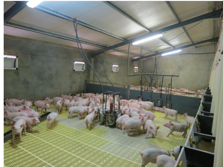
f – Inside a typical weaner room showing drinker system
