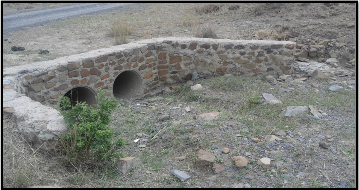
Photograph 3: Showing stone pitched pipe culverts with headwalls.
