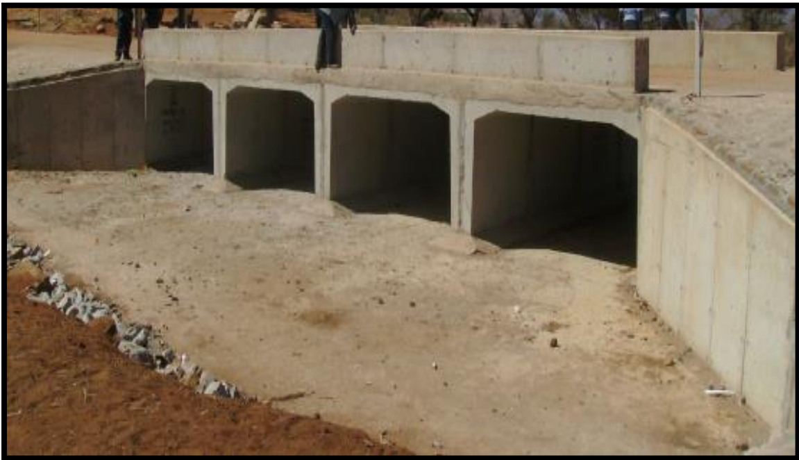
Photograph 1: showing example of a portal causeway structure.
