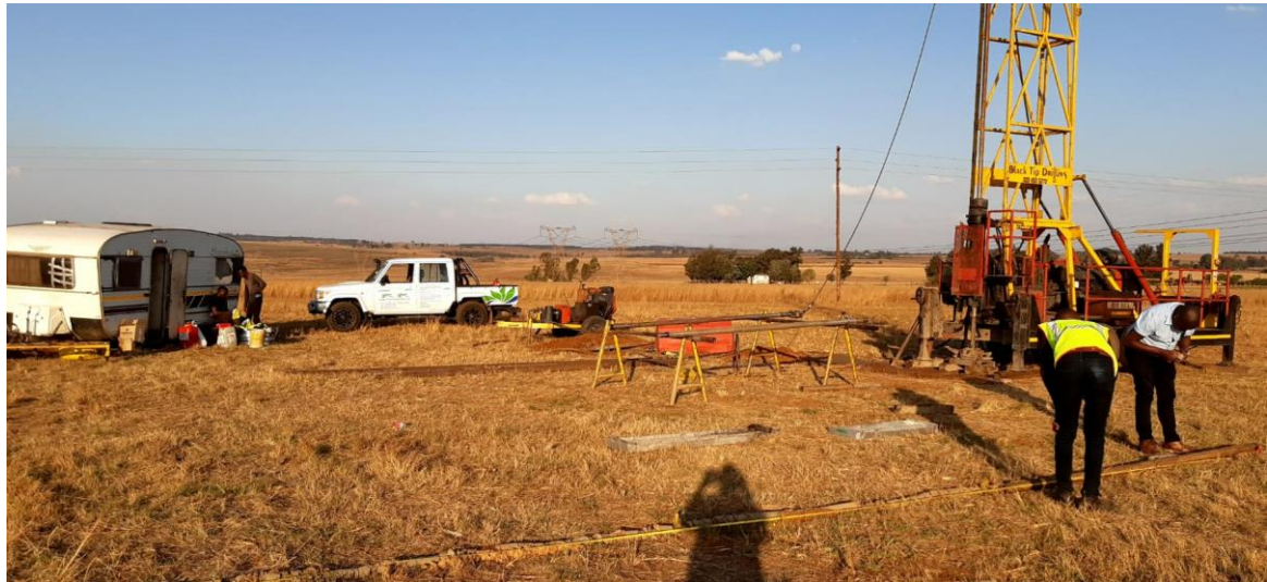
Figure 4: A typical example of diamond core drilling rig.
