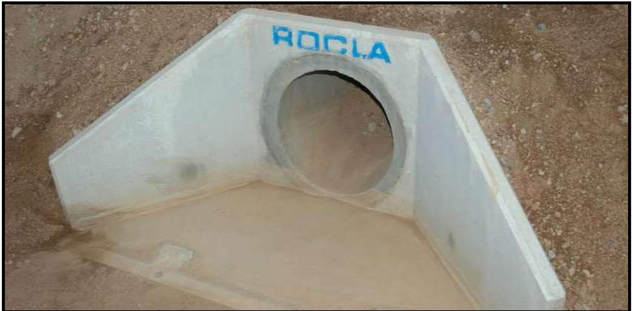
Figure 2: Showing a concrete pipe culvert structure with headwalls.
