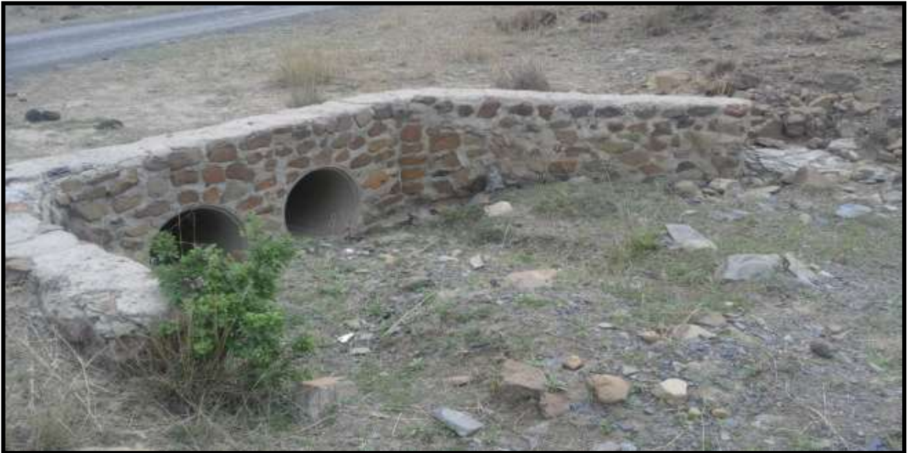
Figure 3: Showing stone pitched pipe culverts with headwalls
