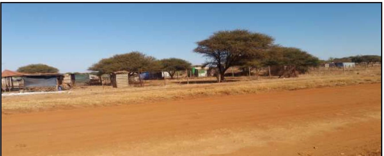
Picture 7: Existing access road
