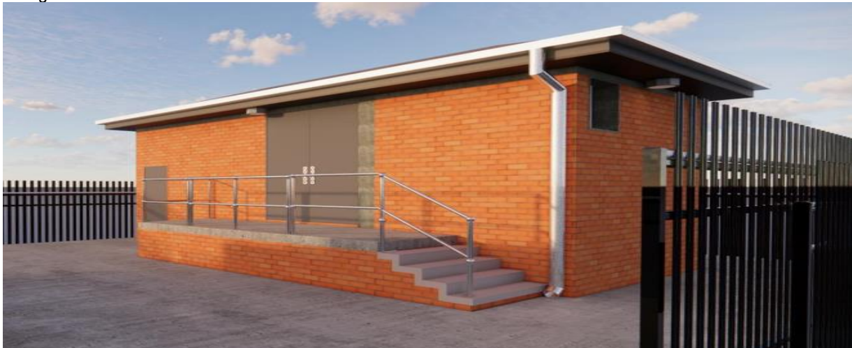
Figure A12: MV Substation (typical)
