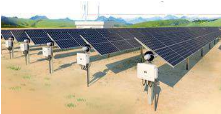
Figure A9: Typical String Inverter installation
