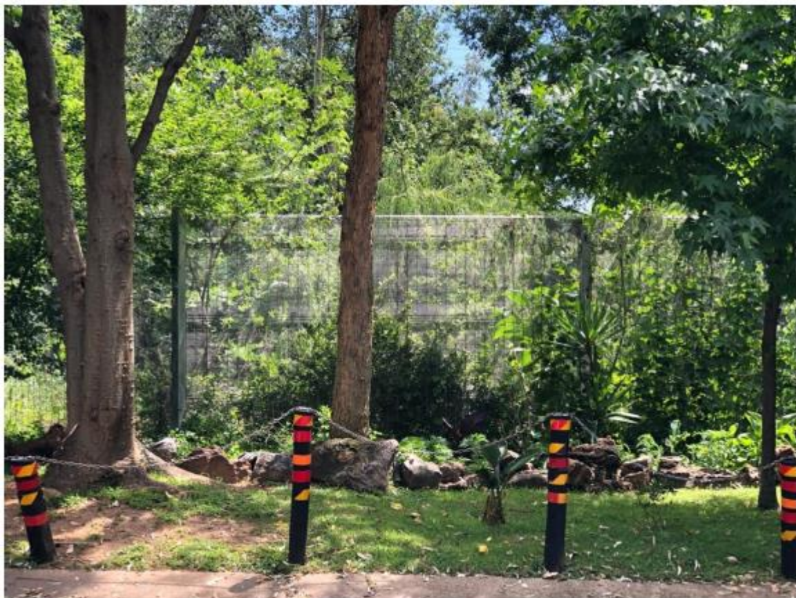
Fig: Example of fencing over river crossing within access controled area.
