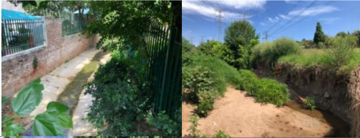
Fig: Left – concrete canal flowing from Main street towards the river. Right – Dry riverbed towards the Braamfonteinspruit.
