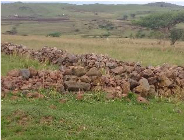
Photo 19: View of old house foundations
