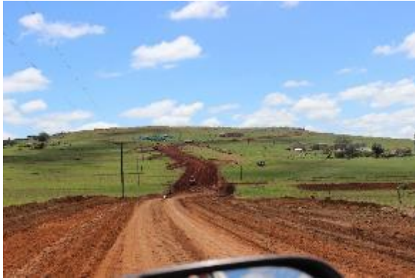
Photo 1: Existing Mantuli track on hilly terrain
