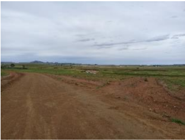
Photo 13: Section of the Road L1970 constructed in the channelled wetland system
