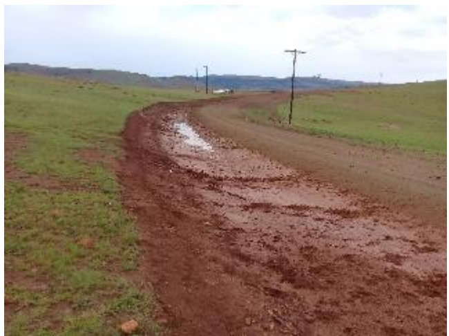
Photo 16: View of clearance of vegetation for road reserve
