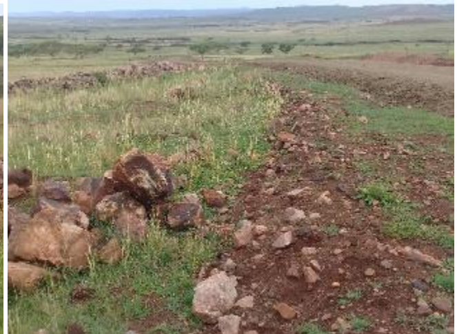
Photo 20: View of damaged old house foundations
