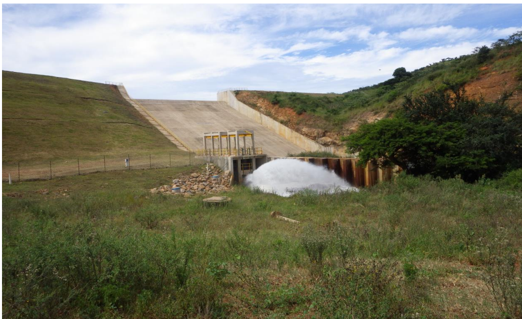
Figure 5: Flow Regulation, Channel and Bed Modification (Site A3; February 2018)
