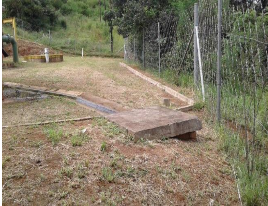
Photo 1: View of the drain and entrance to the outlet pipe of the raw water pumphouse in close proximity to the Imvutshane River.
