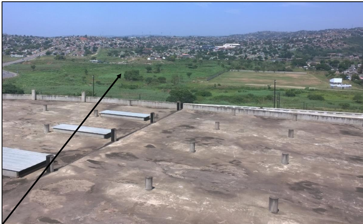
Figure 2: Depicting the aerial view of the proposed BP Service Station construction site from the Bridge City shopping complex, West of the proposed site.
