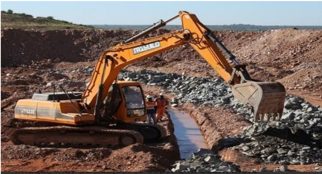
Figure 4.2: Illustration of dirty water trench
