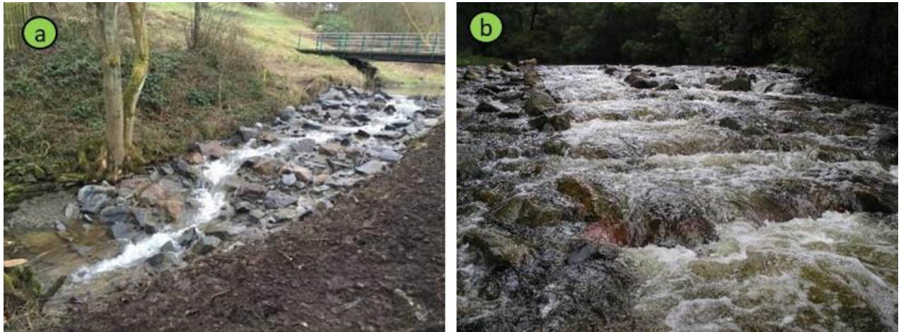
Figure 38 a and b: The aim of a rock ramp type fishway is to simulate a natural rapid-type habitat unit that would allow fish to overcome an otherwise hydraulically difficult area.
