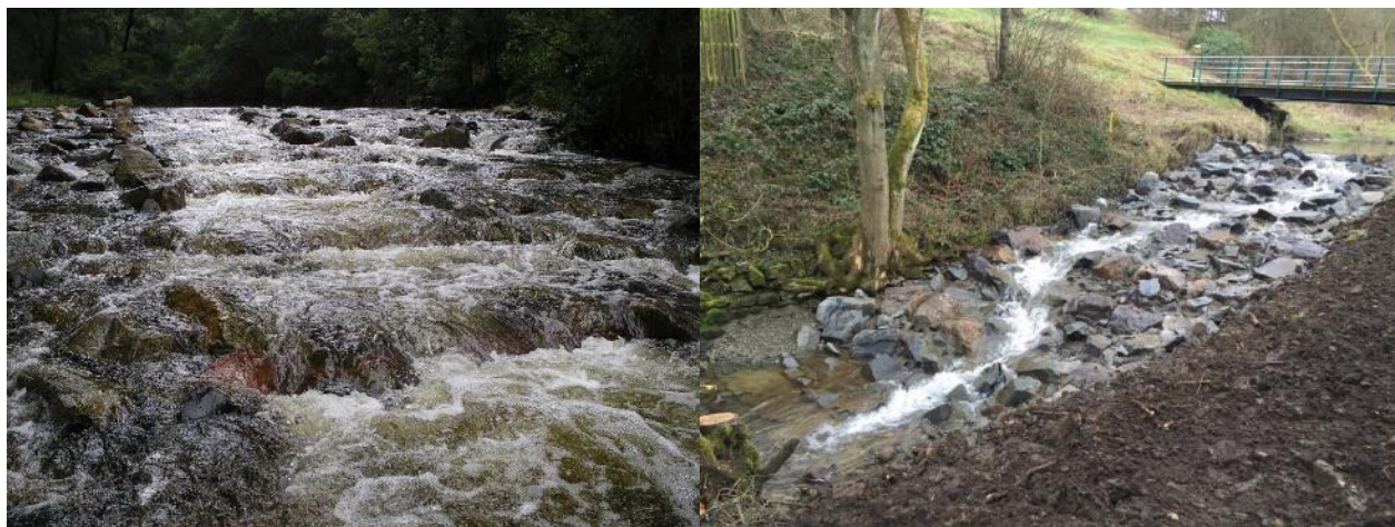
Figure 2: A typical rock ramp fish pass that has made use of embedded boulders to roughly shape consecutive pools. The variable hydraulic conditions are clearly seen, which is a feature that makes the rock ramp fish pass successful in enabling migration of a wide diversity of fish species and size classes.
