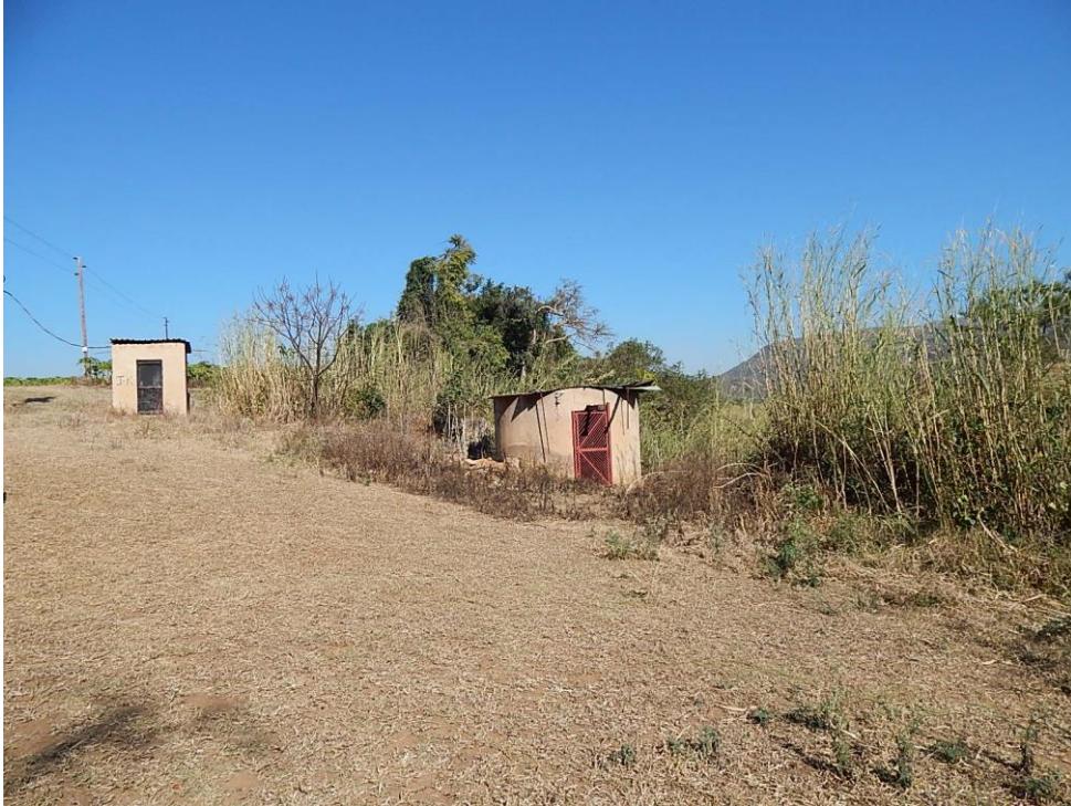
Fig. 5: The section on the western side between the Low's Creek and the Kaap River. Recent pump house structures are visible (farm ESPERADO ANNEX).
