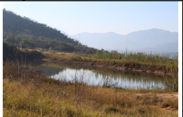
Figure 12: Existing irrigation storage dam on the farm.
