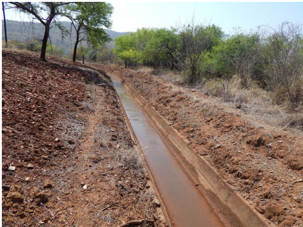
Fig. 42: Another view of the concrete water canal.
