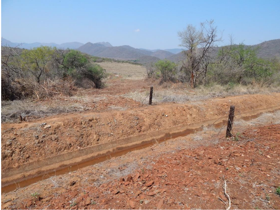
Fig. 41: A concrete water canal cuts through this section in the east. View towards the eastern boundary.
