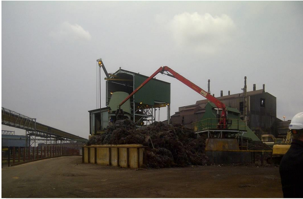
Figure 5: Steel shaving stockpile area showing magnet that loads the shavings onto feeding vibrators
