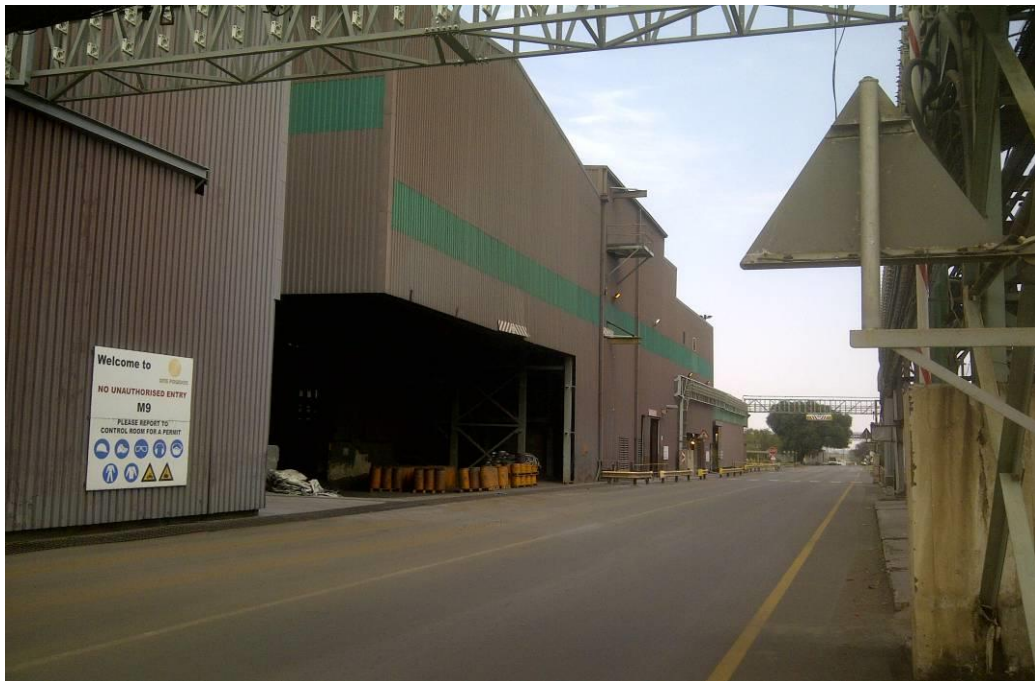
Figure 8: DMS Powders plant (2)
