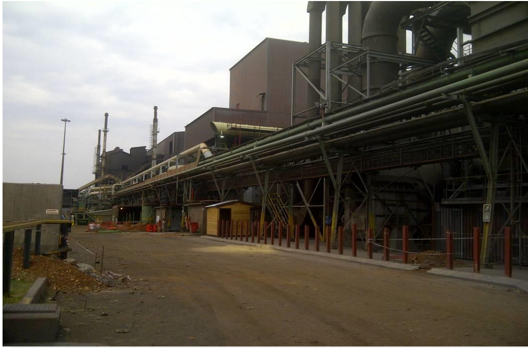
Figure 7: DMS Powders plant (1)
