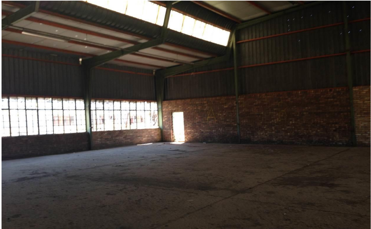
Figure 8: Inside of building 1
