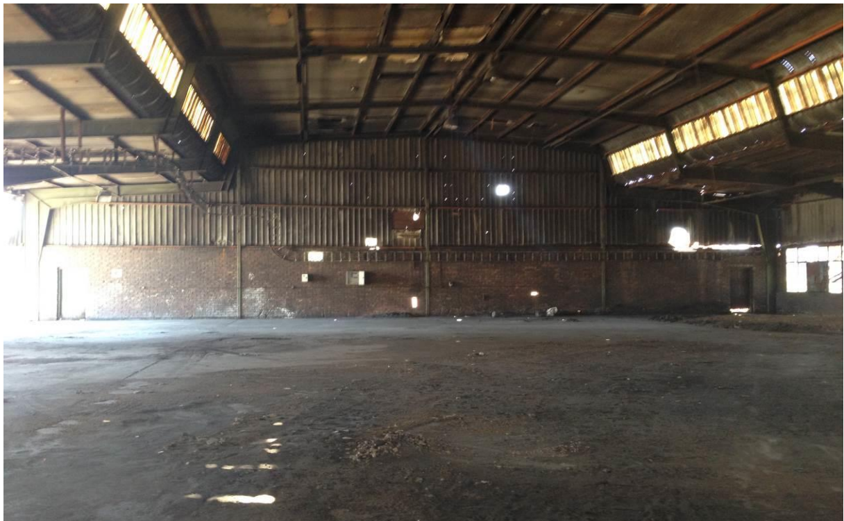
Figure 9: Inside of building 2
