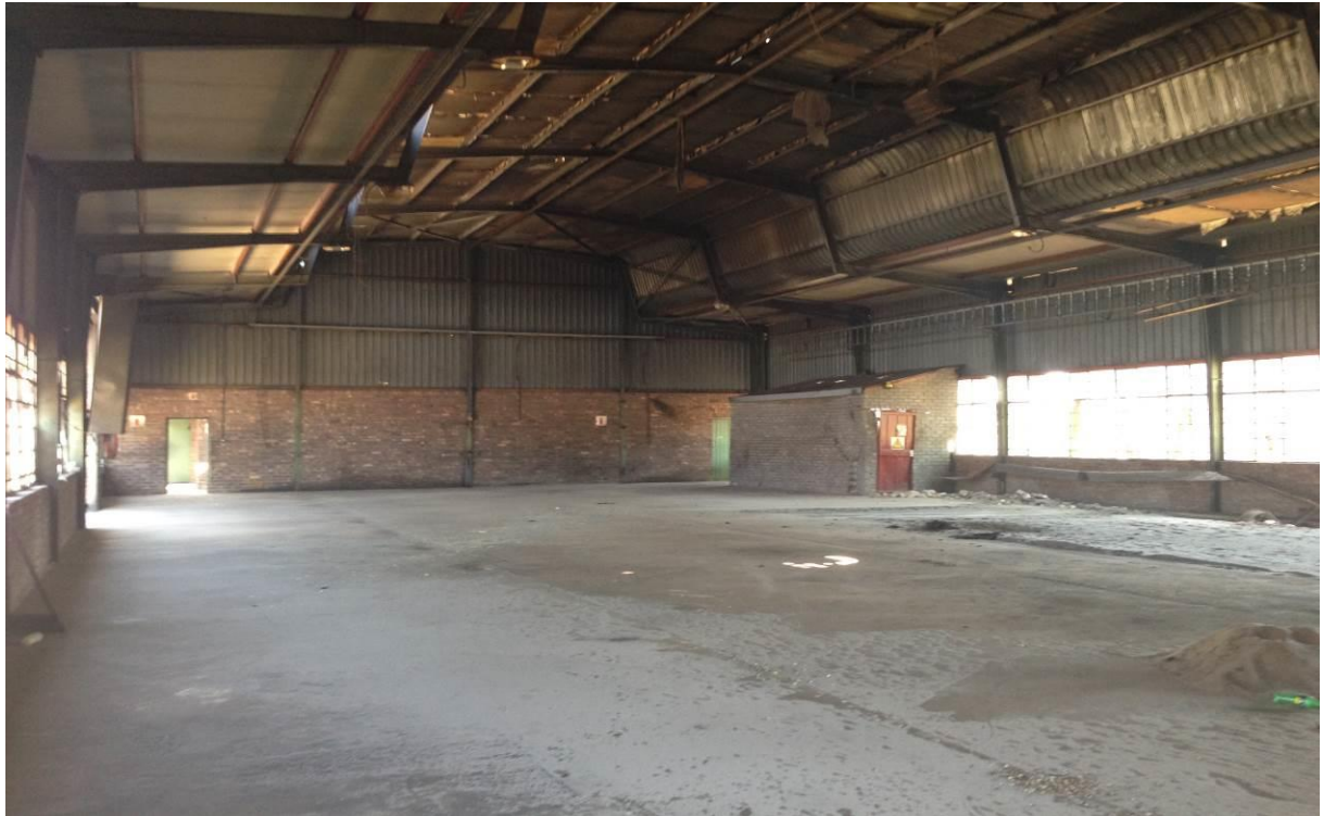
Figure 10: Inside of building 3
