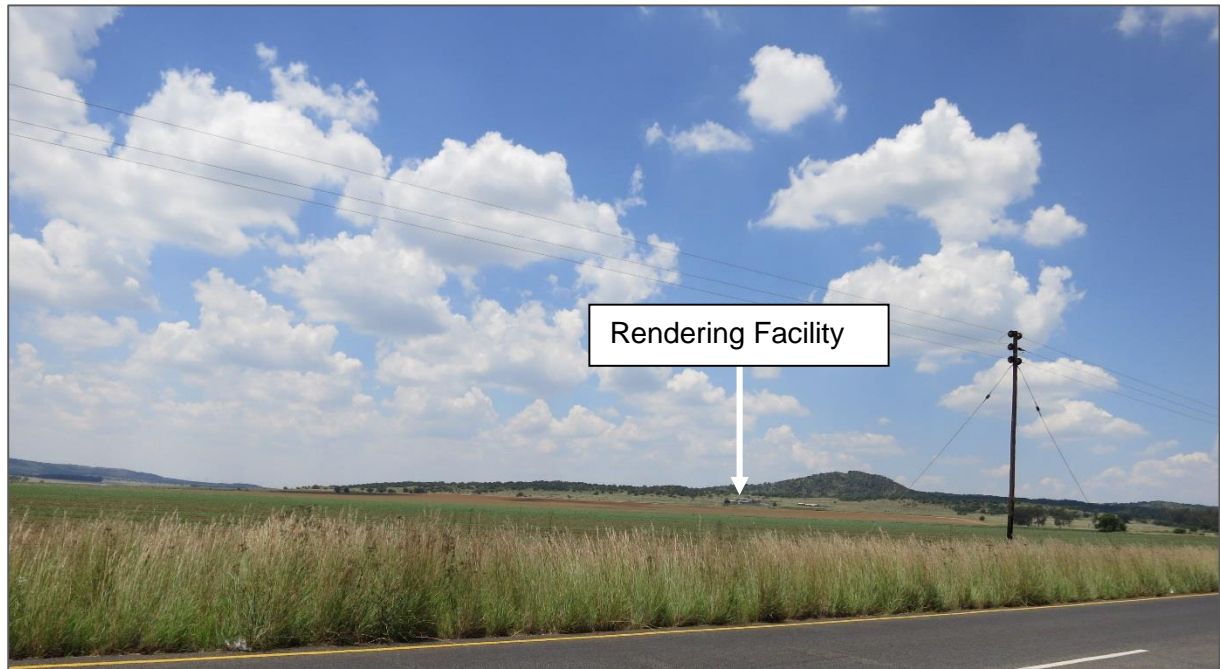
Figure 47: View of the site from the Schoemansdrift Road
