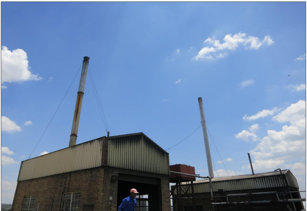
Figure 8: The two boiler stacks
