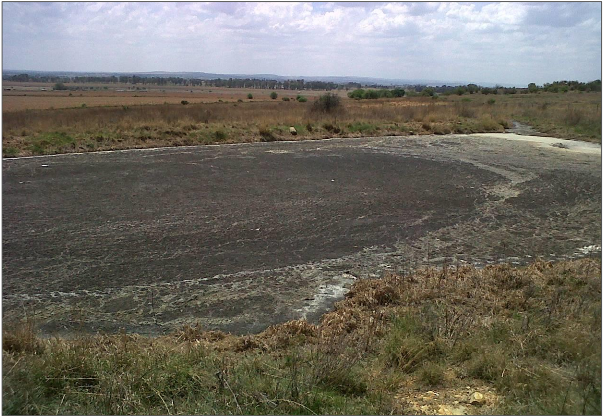
Figure 17: The existing wastewater evaporation pond
