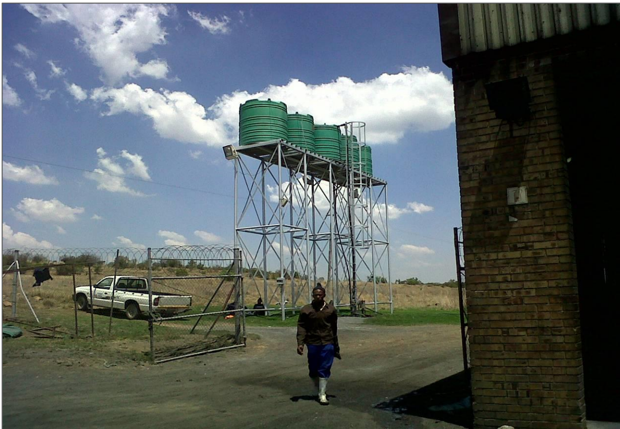
Figure 4: JoJo tanks used to store borehole water from an adjacent property
