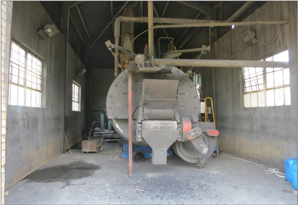
Figure 7: One of two coal fired boilers used to generate steam on site
