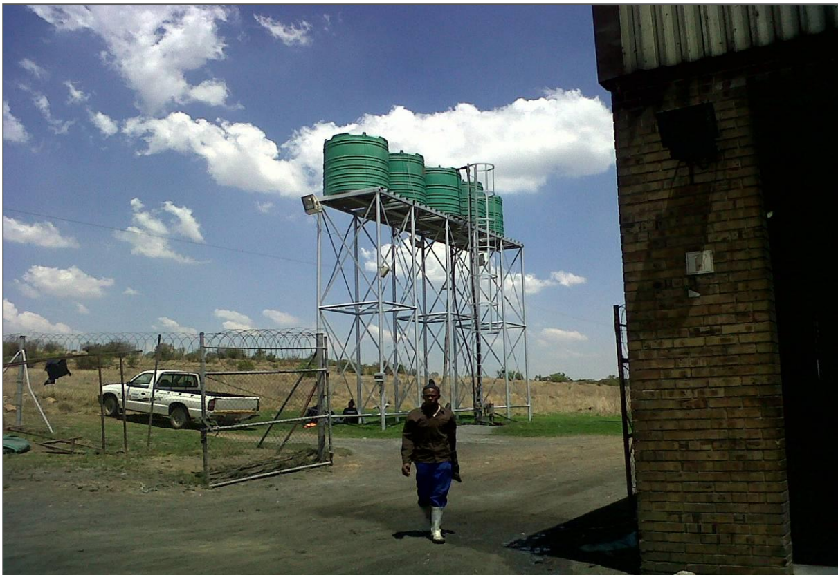
Figure 4: JoJo tanks used to store borehole water from an adjacent property
