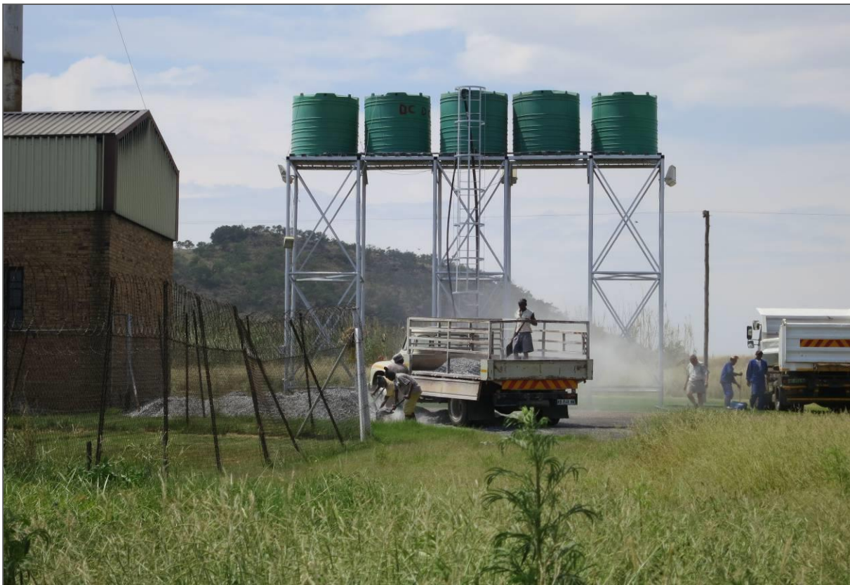
Figure 16: Removal of boiler ash
