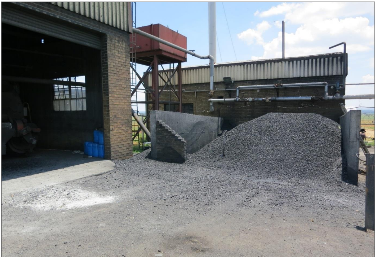
Figure 6: The coal storage bunker
