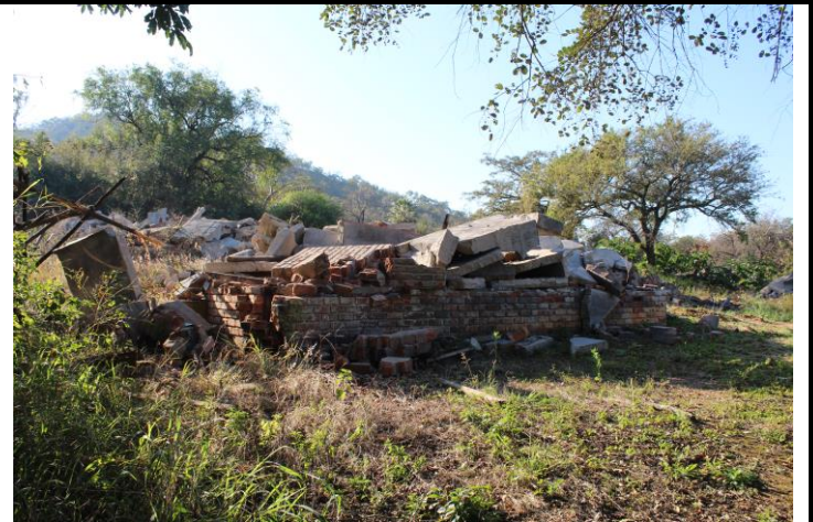
Figure 14: Many buildings have become derelict and the sites will be rehabilitated and become part of the orchards.
