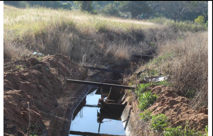
Figure 10: Existing irrigation canal winding through the farm.
