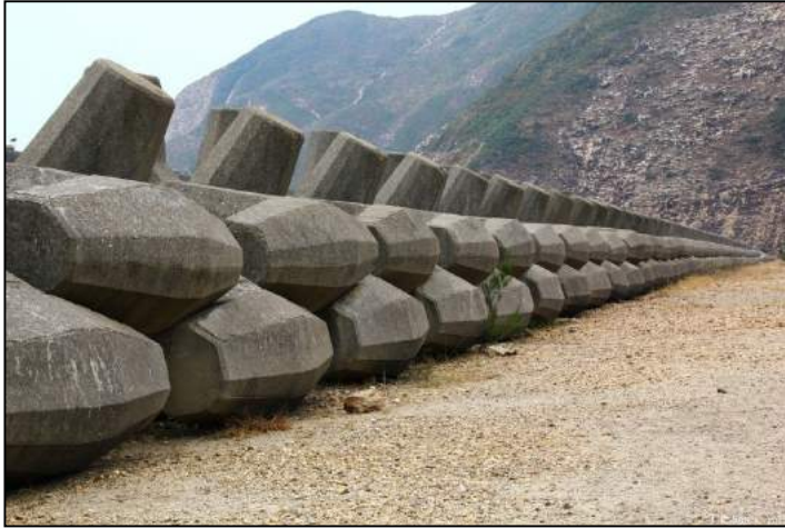
Figure 8-7: Dolosse as an alternative to fencing.
