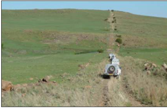
Figure 10-15: Subsurface damming up of the ground water to the left of the road.
