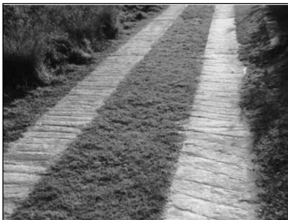
Figure 8-4: Concrete strip pavement on straight sections (Source:C &Ci)
