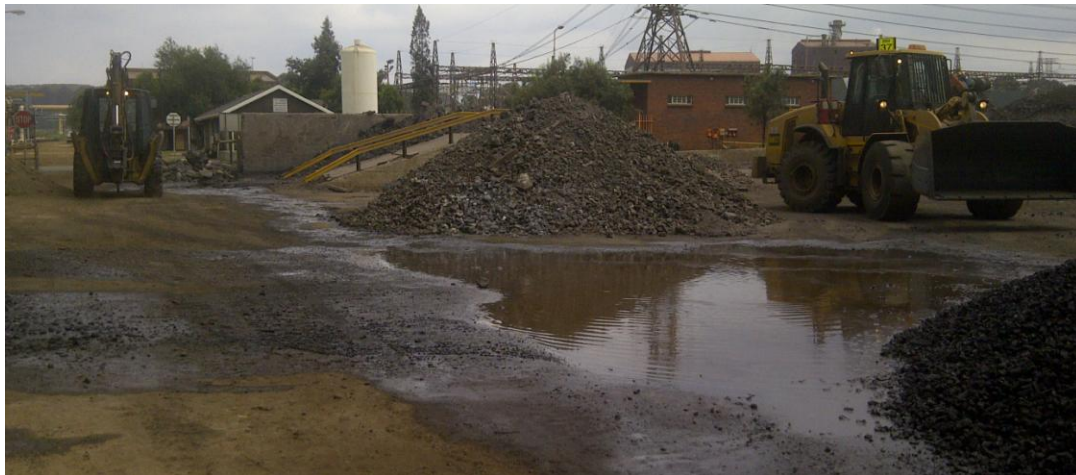
Figure 3: Illustration of steel shaving stockpiles (1).
