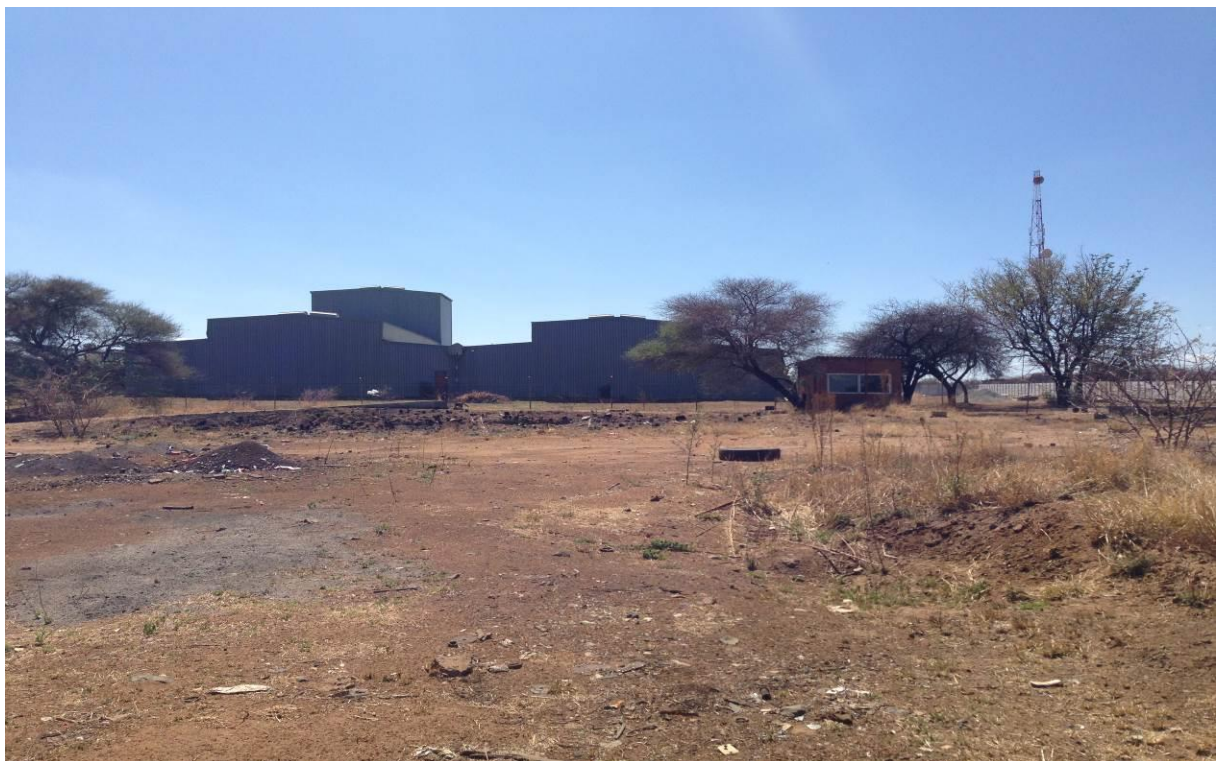
Figure 11: Open piece of land to the east of the three existing buildings (1)
