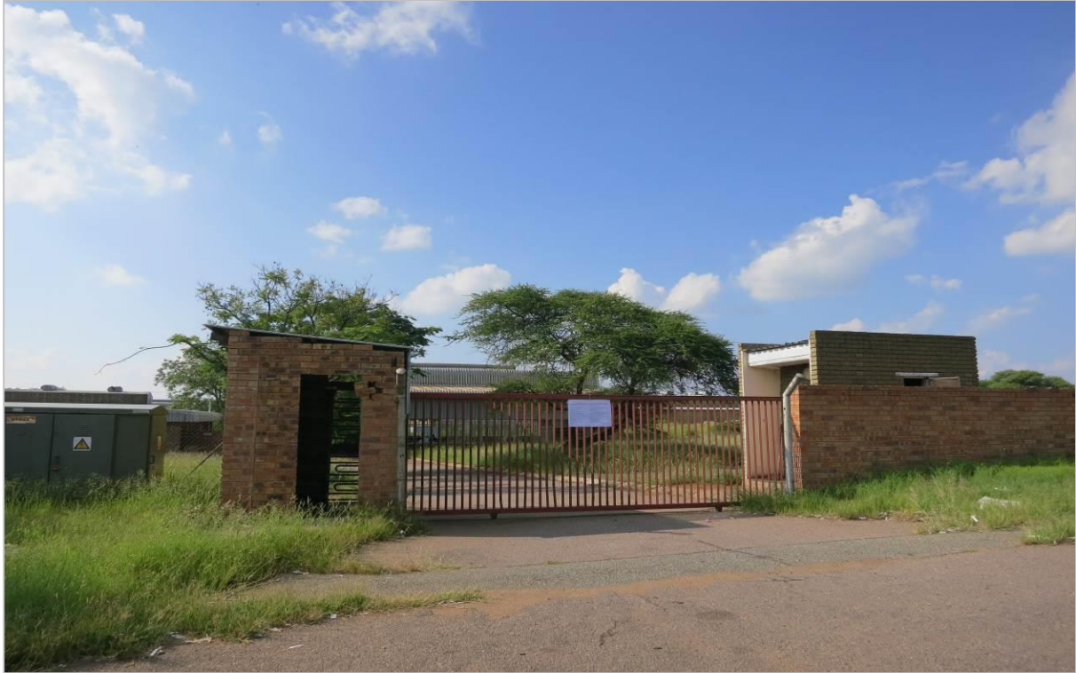
Figure 25: Site notice 1 at the entrance gate to the proposed site
