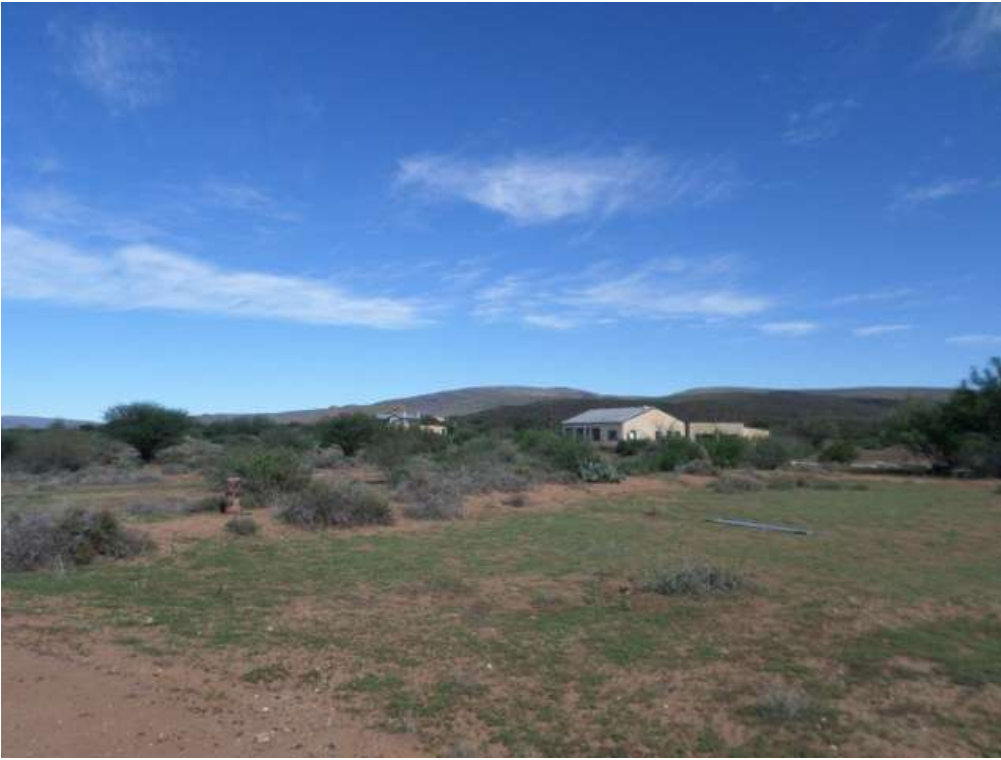
Figure 4: Portion 2 and 4 Rietfontein: Abandoned farm buildings
