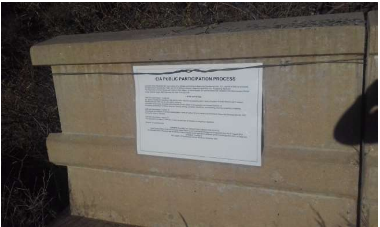
Bridge on Site of Farm Koegas
