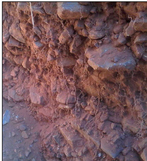
Figure 4: An example of the many plant roots growing within the loose stones layer.
